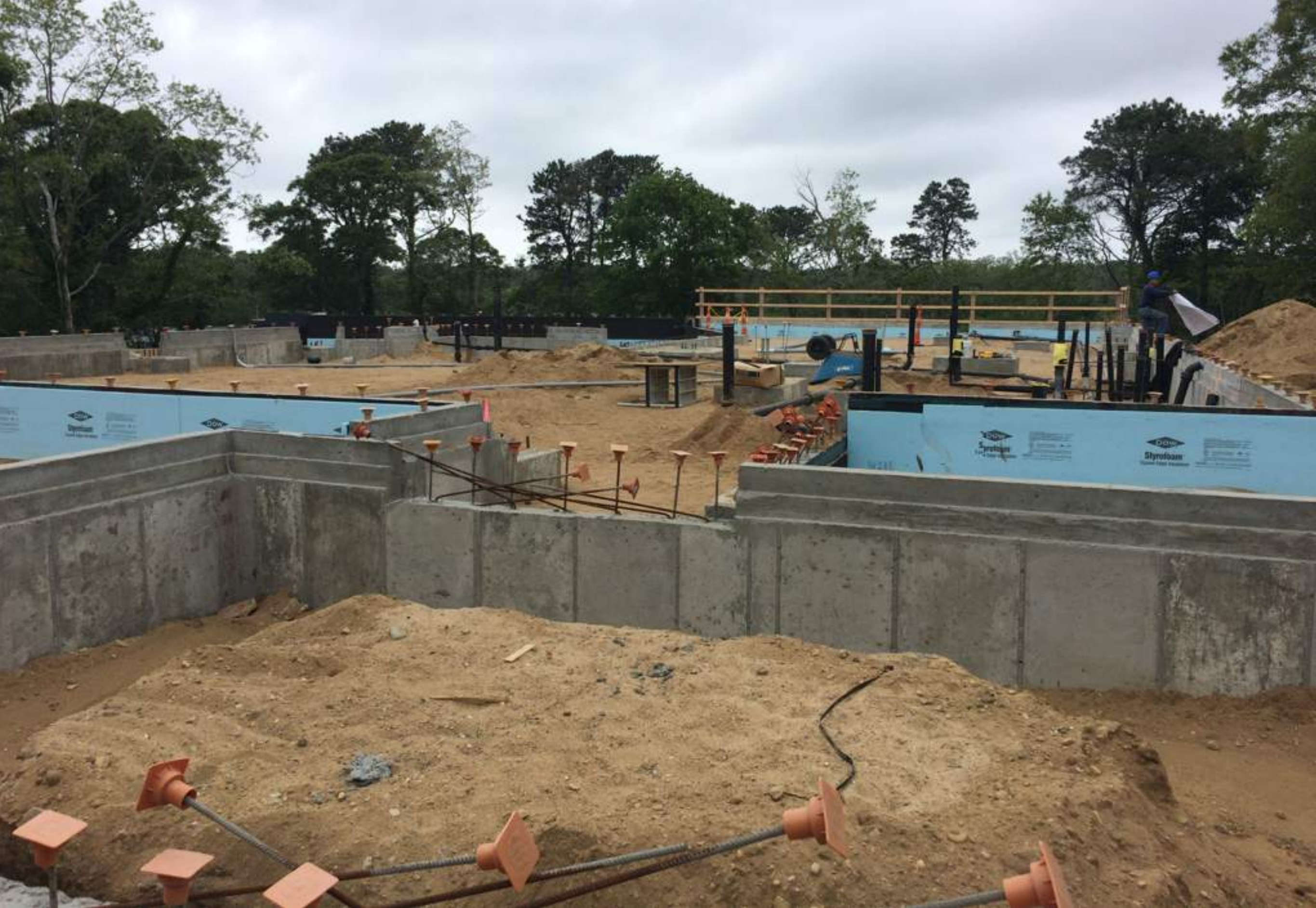
Construction Progress: Under Slab Plumbing
